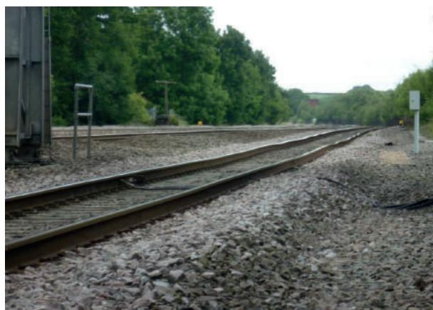
**Figure 2. Intense deterioration of track geometry as a result of low track stiffness**
