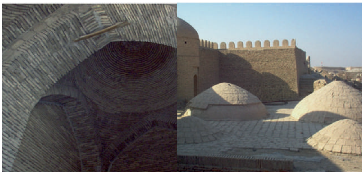
Figure 3. Dome closure at the bottom of the stone gate corridor and the roof ceiling
